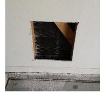
Determine where you want the wall vent and trace the inset frame and drill each corner all the way through the exterior wall. Make the cut in the drywall as drawn.
